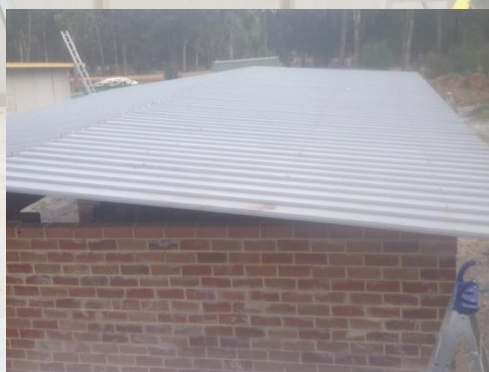
Fast Fix Profiled Roofing used as the roof cover, insulation and ceiling on Brick Walls
