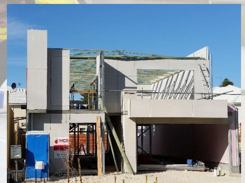
Fast Fix Wall Panels used with a first-level concrete floor and Timber-Framed Roof
