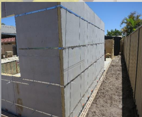
Fast Fix Single Wall being used as the internal leaf in a brick cavity system
